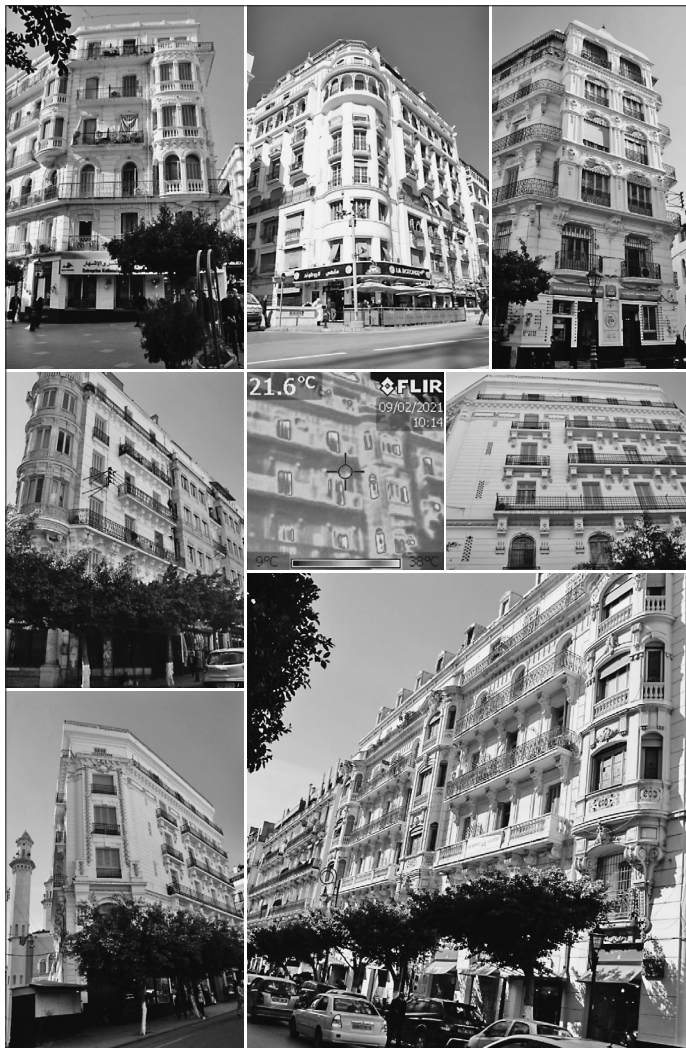
FIG. 1 REPRESENTATIVE BUILDINGS WITHIN THE LARBI BEN M'HIDI DISTRICT, ALGIERS. (SOURCE: AUTHORS, 2025)
