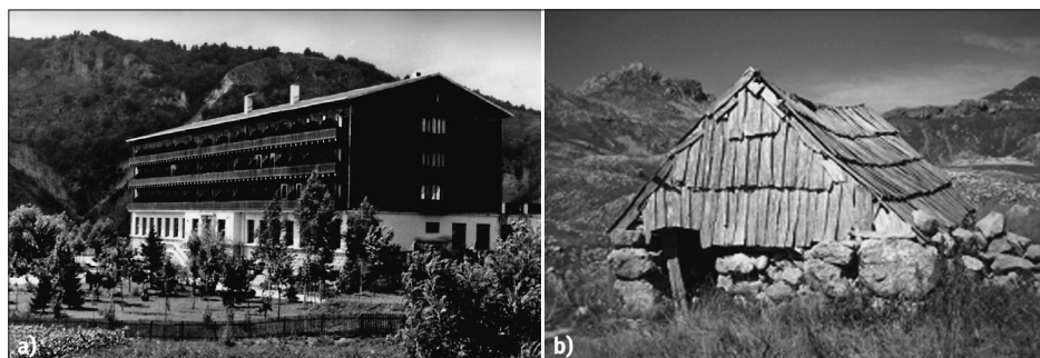
FIGURE 7 A. ORIGINAL BJELASICA HOTEL PRIOR TO ZEKOVIC'S INTERVENTION; B. TRADITIONAL HOUSE IN THE BJELASICA HIGHLAND SETTLEMENT
