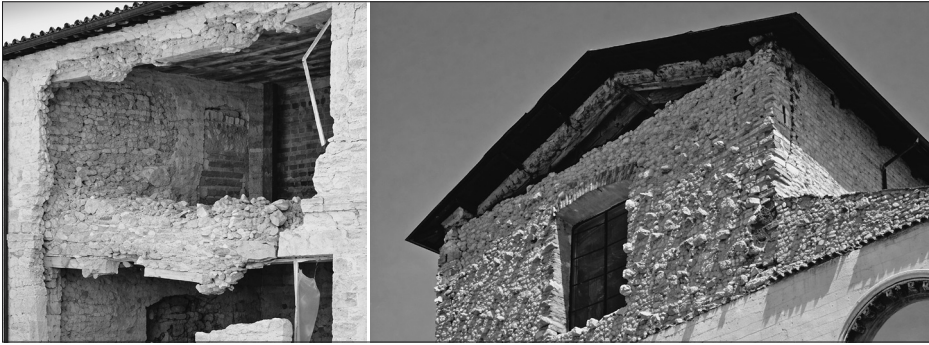
FIG. 2 INADEQUATE STRENGTHENING METHODS (BINDA AND MODENA, 2011)
