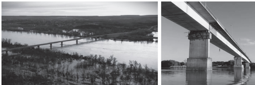
Figure 1. Ilok - Bačka Palanka bridge
