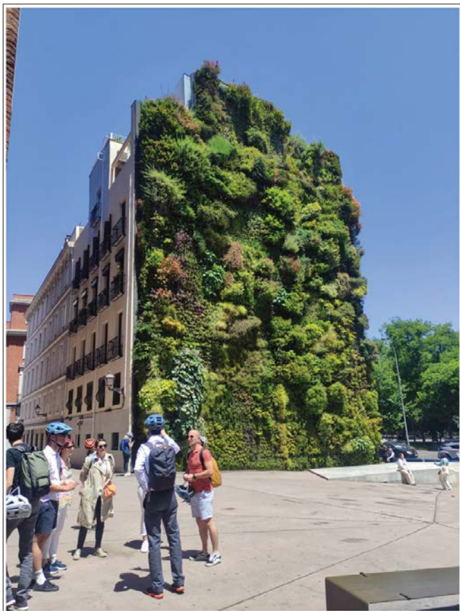
Figure 3. Green wall integrated into a building façade as a vertical greening system, increasing structural habitat complexity and contributing to urban ecological infrastructure by supporting insect habitat availability in densely built environments (Ivana Pajač Živković, Madrid, Spain)
