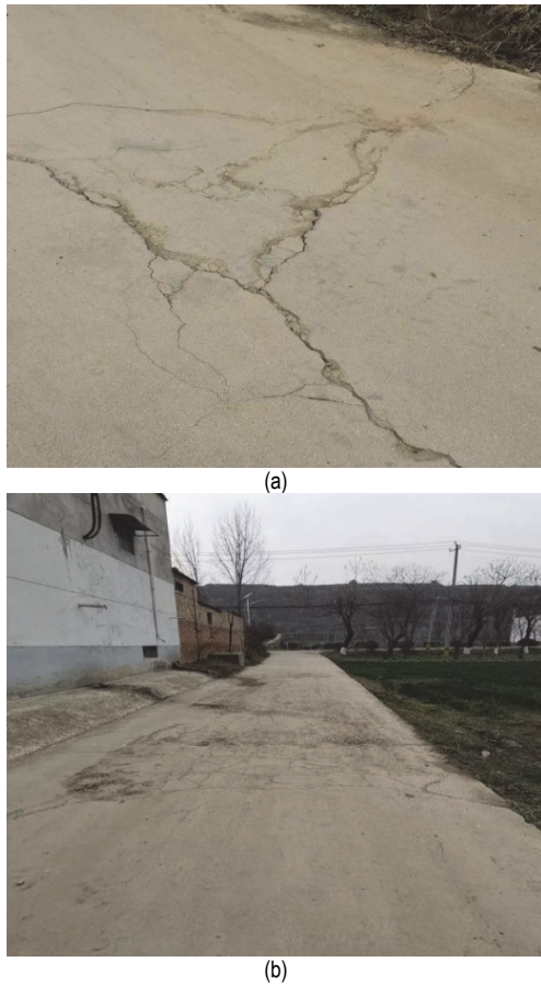
Figure 10 Road conditions in Zuitou Village
