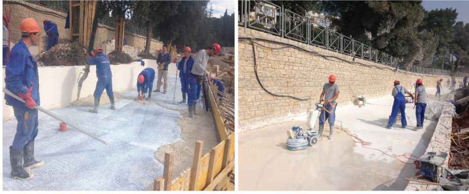
Fig. 11: Placing of white concrete (left) and final grinding and polishing (right).
