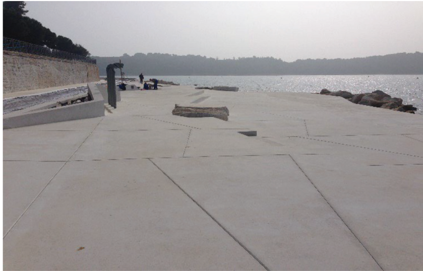
Fig. 12: View of the promenade and beach, constructed using white concrete.
