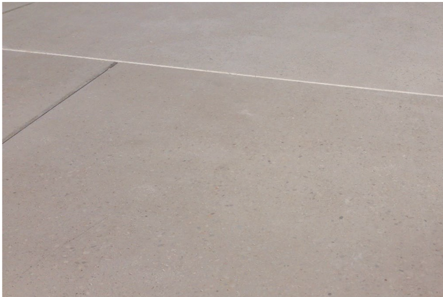
Fig. 10: Final visual appearance of grinded white concrete surface.
