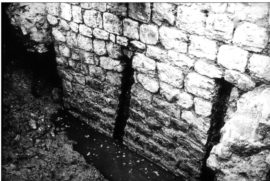
Figure 7. Remains of a bridge-tower, exterior
