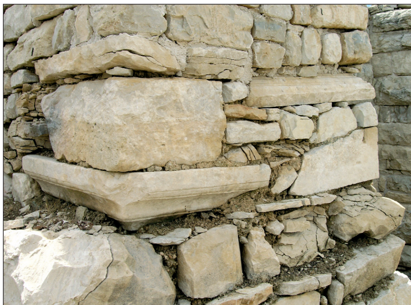
Sl. 17. Dio are unutar strukture prvoga kasnoantičkoga kontrafora Fig. 17. Fragment of the ara within the structure of the first late Roman buttress
