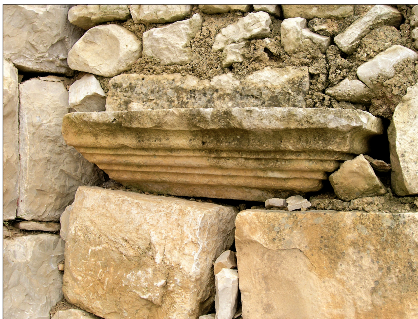
Sl. 11. Kruništa are unutar strukture prizidane kasnoantičke kule Fig. 11. Crown of the ara within the structure of the late Roman turret
