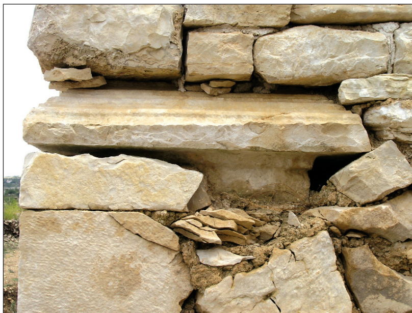
Sl. 16. Krunište are unutar strukture prvoga kasnoantičkoga kontrafora Fig. 16. Crown of the ara within the structure of the first late Roman buttress
