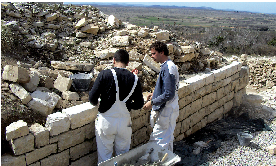
Sl. 3. Konzervatorsko-restauratorski zahvati na prednjem dijelu zapadnih vrata (južni zid) Fig.3. Conservation and restoration on the frontal section of the western gate (southern wall)
