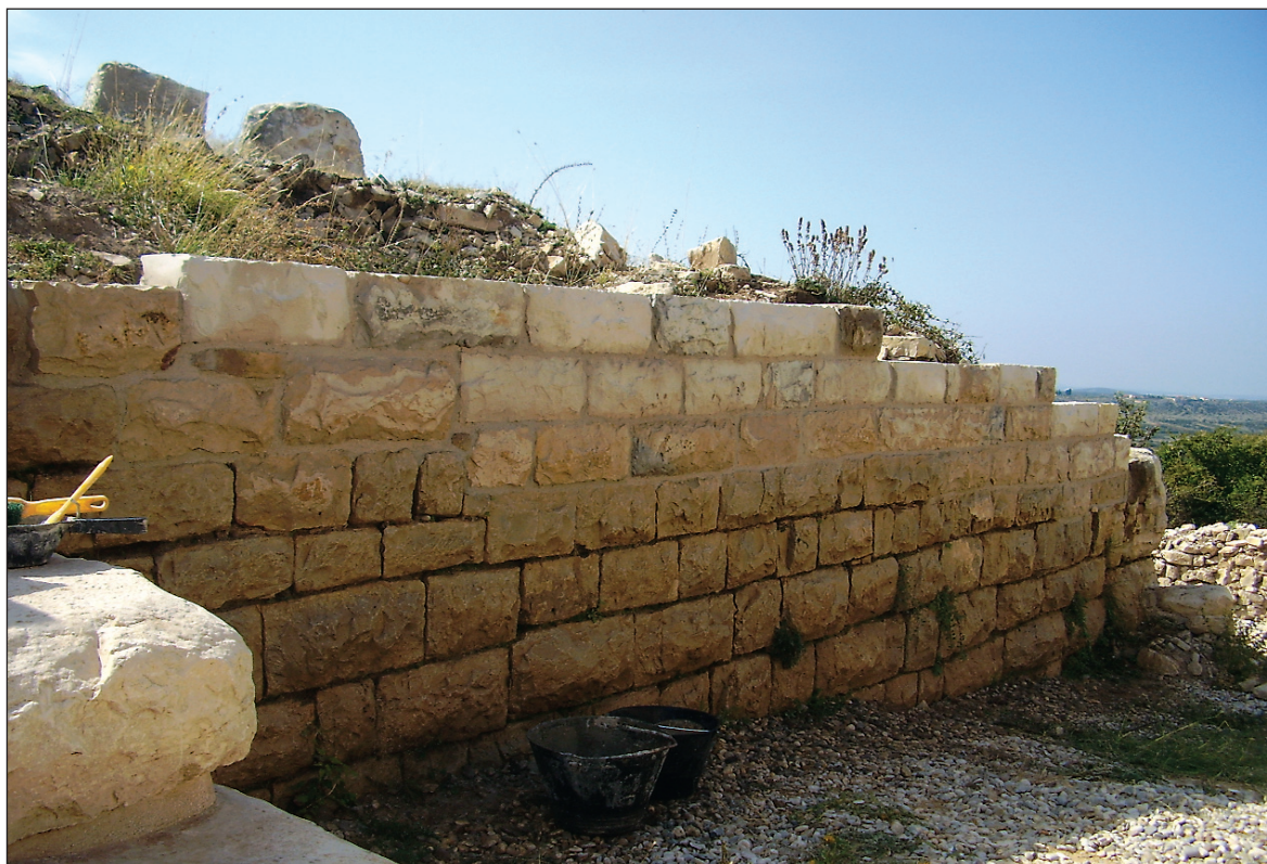
Sl. 5. Pogled na prednji dio južnog zida zapadnih vrata - završeni konzervatorsko-restauratorski radovi Fig.5. View of the frontal section of the southern wall of the western gate – after the conclusion of conservation and restoration
