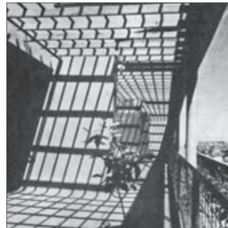
SL. 23. VIŠESTAMBENA ZGRADA, ULICA GRADA VUKOVARA 35-35A, DETALJ TERASE S BETONSKOM 'MREŽOM' FIG. 23 APARTMENT BUILDING, 35-35A VUKOVAR STREET, TERRACE DETAIL WITH CONCRETE 'GRID'
