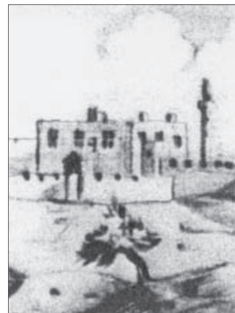
FIG. 22 ILOK, TOWNSCAPE BY S. SCHMALKALDER, DESTROYED PALACE OF THE PRINCES OF ILOK, DETAIL
