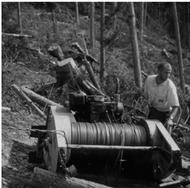
Figure 3 Gantner cable crane
