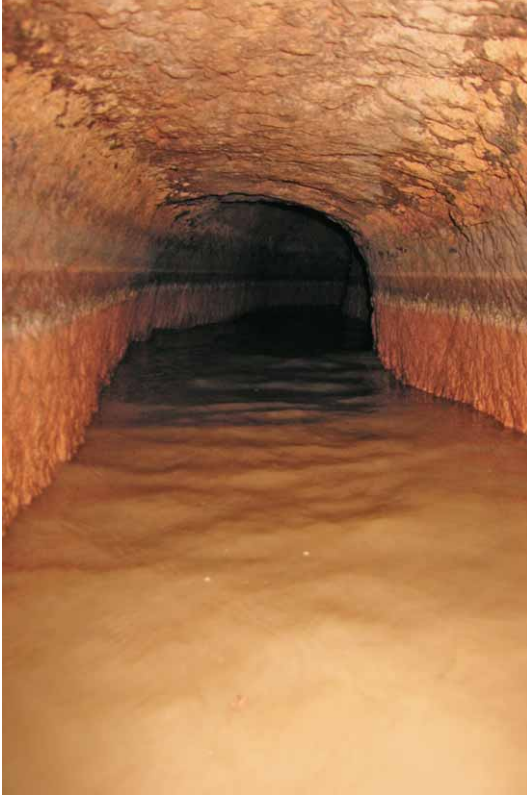
Fig 27 – View into the tunnel beyond the retention (Croatian Conservation Institute – University of Zadar, 2007).
