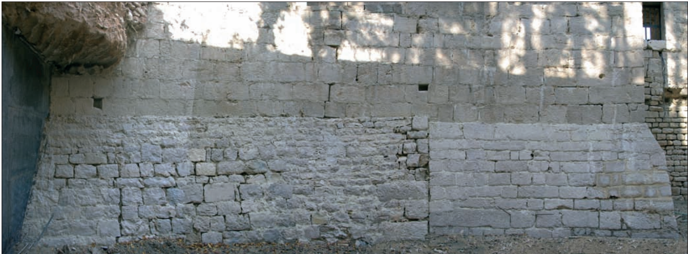
Sl. 8 Pokos na istočnoj strani kule Fig. 8 Batter on the eastern side of the tower
