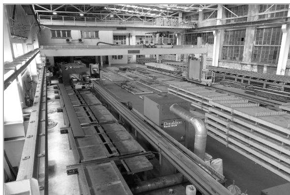
Figure 2. Installed new robotised profile cutting line (source: Shipyard "3.MAJ")
