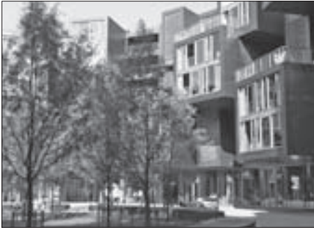
FIG. 9 ØRESTAD, HABITATION HALL (TJETGENKOLLEGIET), ARCHITECTS BOJE LUNGAARD AND LENE TRANBERG, 2006 SL. 9. ØRESTAD, STAMBENI HAL (TJETGENKOLLEGIET), ARHITEKTI LUNGAARD B. I TRANBERG L., 2006.
