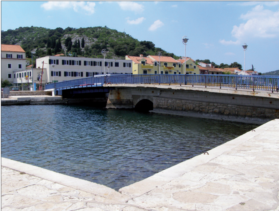
Slika 1. Most u Tisnom (kopno – otok) Figure 1 Tisno, bridge (mainland – island)
