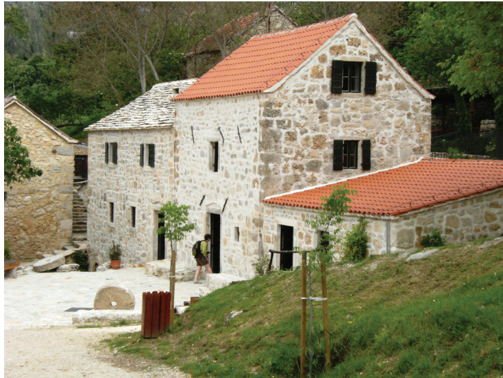
Sl. 3.06. Obnovljena mlinica/Restaurated mill.
