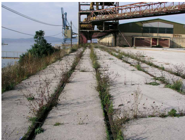
Fig. 1. Gaženica cargo port (Zadar), bulk-cargo reloading dock
