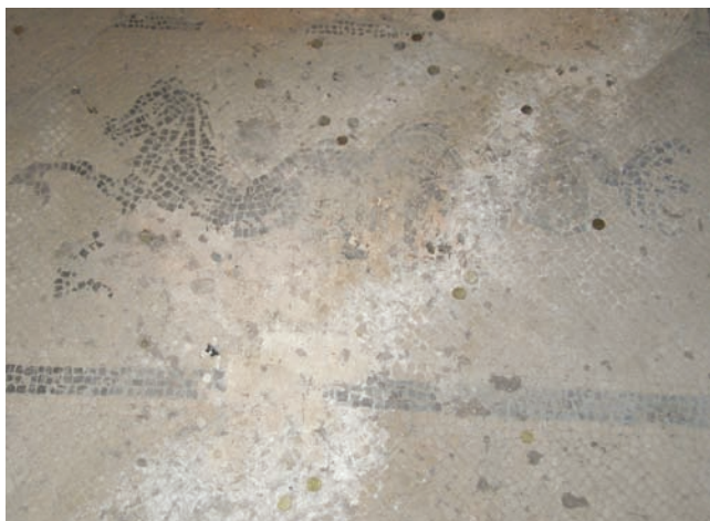
Sl. 4 Motiv hipokampa s vidljivim nakupinama razarajućih soli. Fig. 4 A hippocamp motif with visible accumulations of deleterious salts
