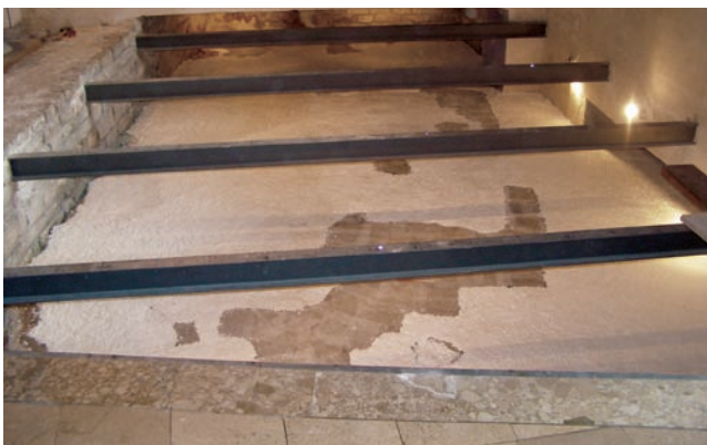
Sl. 11 Stanje mozaika s celuloidnom pulpom nakon restauratorsko-konzervatorskih radova 2009. Fig. 11 The state of the mosaic with the installed cellulose pulp layer after the restoration-conservation works performed in 2009.
