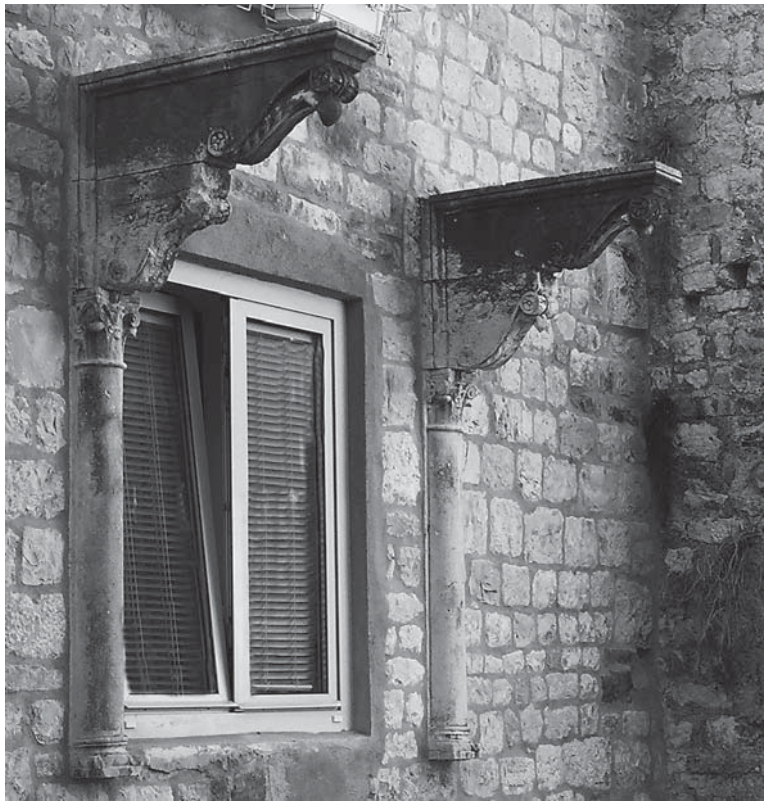
Ostatci kamina Palače Andreis u Trogiru Andreis palace in Trogir, remains of the fireplace
