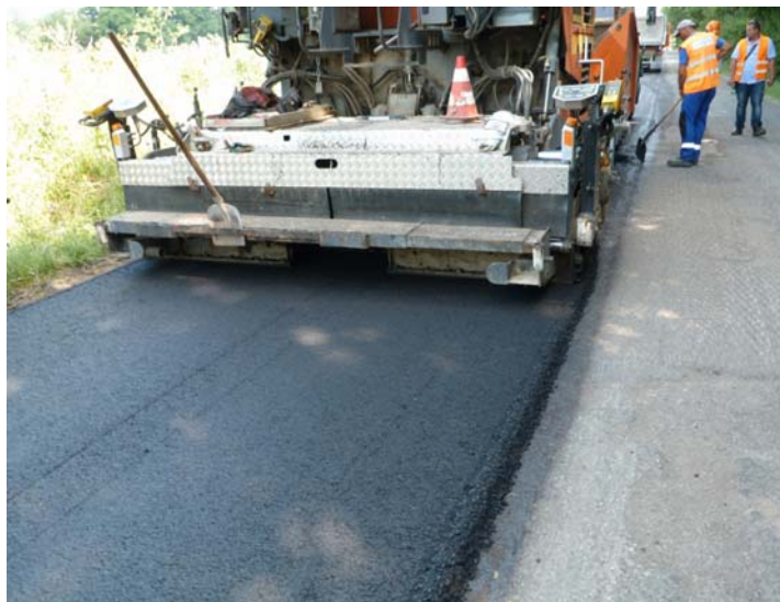
Figure 2. Laying the surface course
