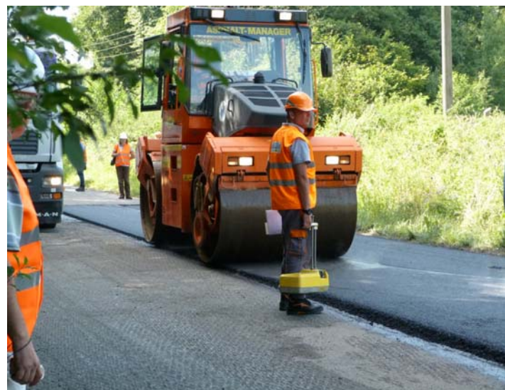
Figure 3. Compacting the layer and density control
