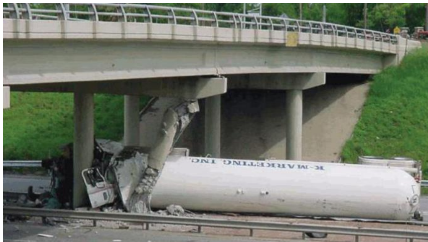
Figure 1 Impact between vehicle and column (U.S. highway) [8]
