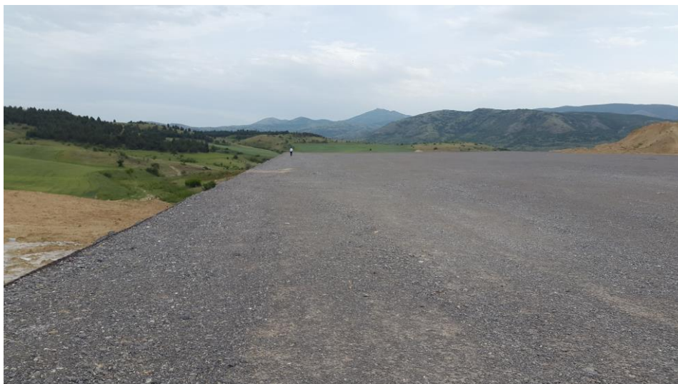
Figure 13 Working platform after construction of RSRW
