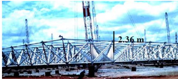
Figure 2 Trusses bolted on the ground [3]
