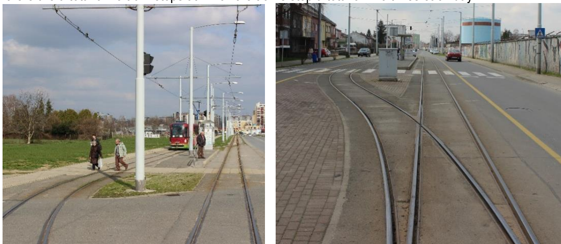
Figure 5 Passing loops with tram stops on Line 2
