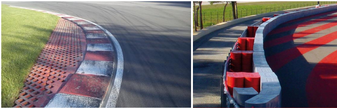
Figure 6 Inner curbs and TECPRO energy dissipation system [16, 17]
