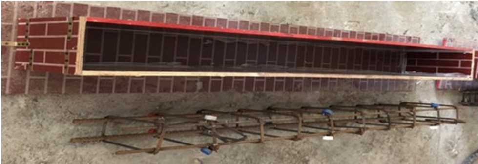
Figure 8. Wooden moulds for beams
