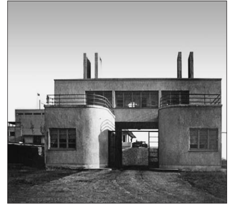
FIG. 5 ÇUBUK DAM WATER FILTERING STATION
