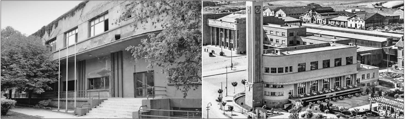
FIG. 4 ANKARA TRAIN STATION MUSIC HALL: VERTICAL BANDS OF ORNAMENTATION AND METAL RAILINGS (LEFT)
