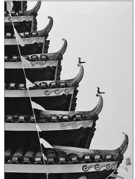
FIG. 9 THE UPTURNED EAVES ARE DECORATED WITH BIRD FIGURES (SANJIANG, 2022)
