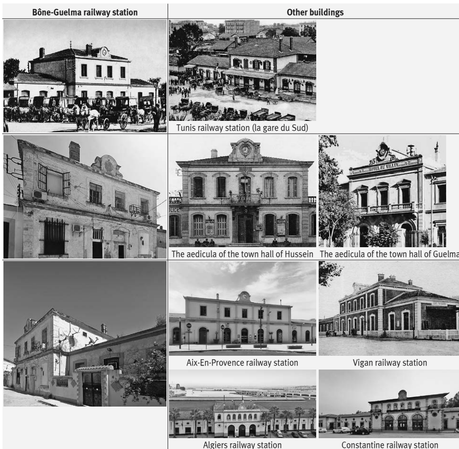
FIG. 7 COMPARISON BETWEEN BÔNE-GUELMA STATION AND OTHER STRUCTURES BUILT DURING THE SAME ERA
