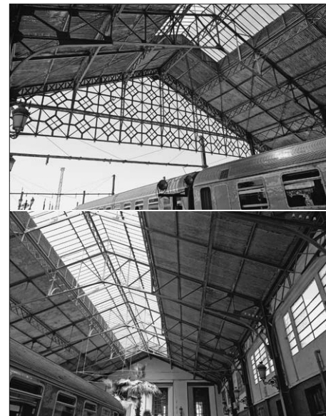
FIG. 15 VIEWS OF THE TRAIN SHED OF BÔNE STATION
