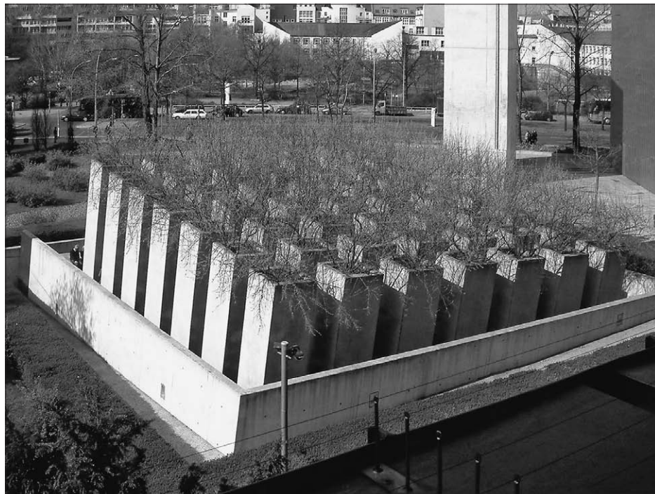
FIG. 5 THE TILTED CONCRETE STELAE AND THE VEGETATION GROWING WITHIN
