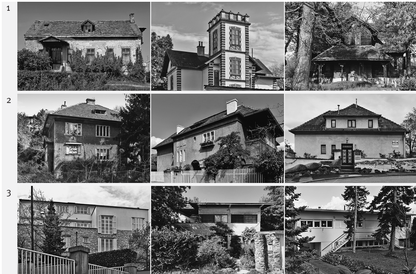
FIG. 1 COMPARATIVE DISPLAY OF RECENT EXTERIOR PHOTOGRAPHS OF SELECTED RESEARCHED BUILDINGS FROM DIFFERENT HISTORICAL STYLISTIC PERIODS (FROM LEFT TO RIGHT): 1 ST HISTORICAL-STYLE PERIOD: SUMMER RESIDENCE TKALČIĆ, SUMMER RESIDENCE VESELJAK, SUMMER RESIDENCE VILLA OLGA 2 ND HISTORICAL-STYLE PERIOD: NASTA ROJC SUMMER RESIDENCE, CITY VILLA VRBANIĆ, HOUSE ŠENOVA 3 RD HISTORICAL-STYLE PERIOD: VILLA MEIXNER, VILLA PFLÜGER, VILLA ALEXANDER
