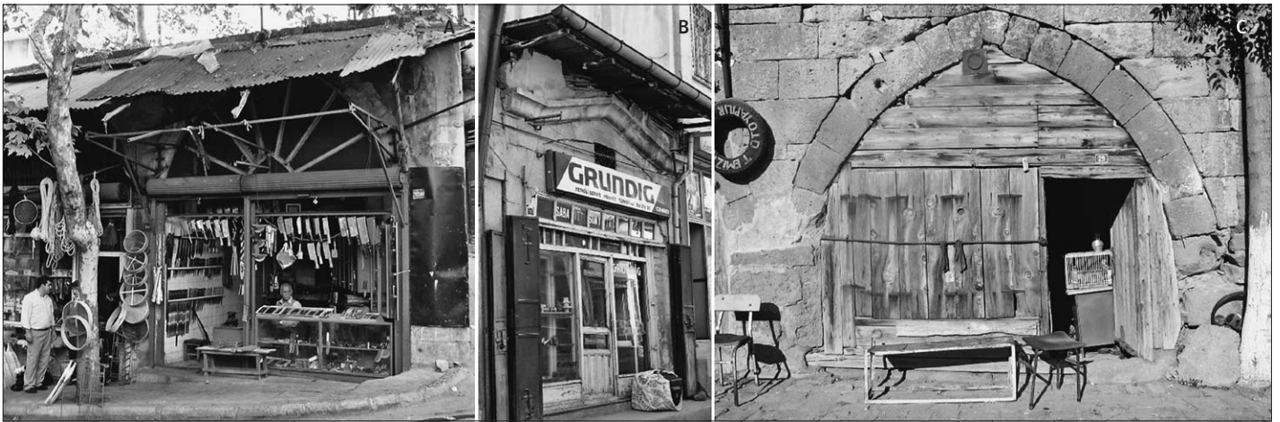
FIG. 9 SHOPS: A – A SHOP FACADE IN MARAŞ BAZAAR; B – A SHOP FACADE IN BEYPAZARI BAZAAR, ITS METAL SHUTTERS WERE FOLDED AT BOTH SIDES; C – TIMBER SHUTTER OF A SHOP IN İNCESU ARASTA
