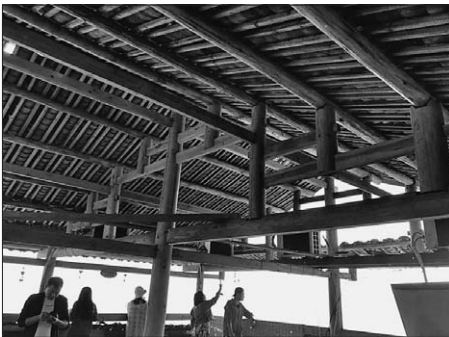
FIG. 7 WOODEN PILLARS OF VARYING LENGTHS IN THE DONG BUILDING (SANJIANG, 2022)
