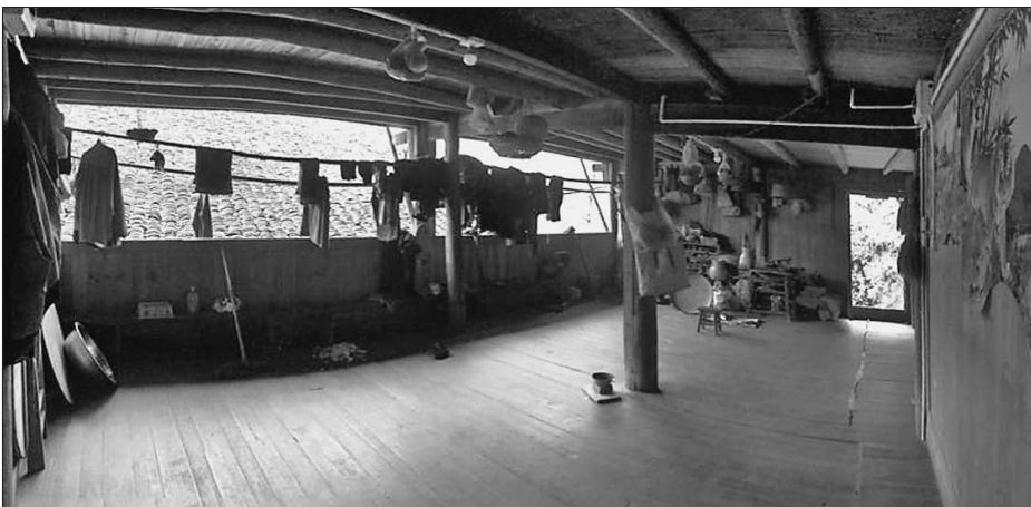
FIG. 8 RESIDENTIAL HOUSE BALCONY (SANJIANG, 2022)
