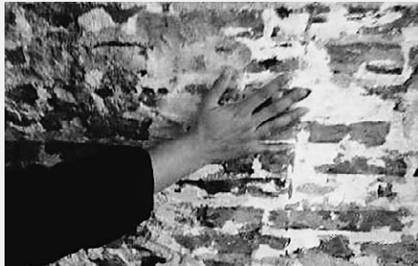
Gypsum plastered stone wall: rough, warm, natural (space 2)
