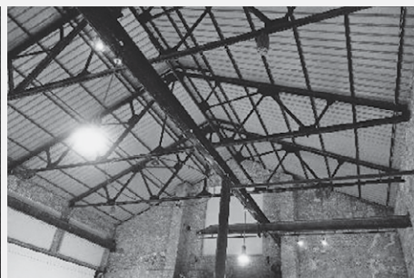
12. Ceiling of the entrance hall: high, rusty, historic
