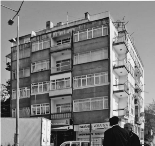
FIG. 1 TYPICAL MID-RISE RC BUILDINGS ENCOUNTERED WITHIN TURKEY'S URBAN PATTERN AND THE RESULT OF EARTHQUAKE DAMAGE IN THE FORM OF TOTAL OR PARTIAL COLLAPSE
