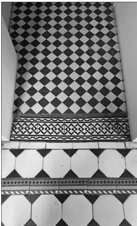
FIG. 8 ORIGINAL FLOOR TILING ON THE SECOND FLOOR
