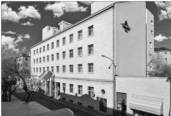
FIG. 3 ANTE BARAĆ: POST OFFICE, SPLIT, MAIN FACADE IN ZAGREBAČKA STREET, 1929-1939
