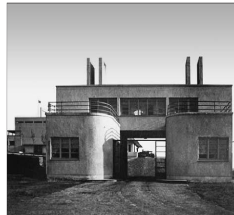
FIG. 5 ÇUBUK DAM WATER FILTERING STATION
