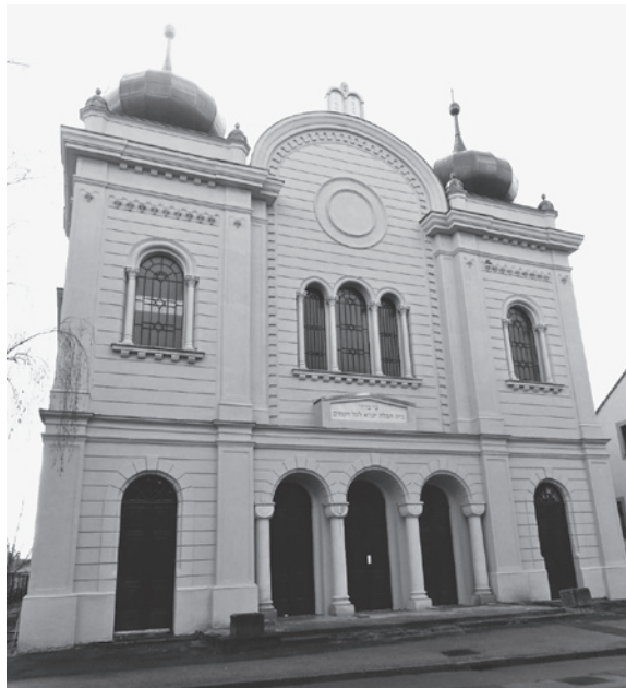
Varaždin Synagogue after the renovation in 2021 19
