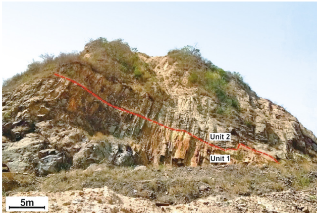
Figure 2: Outcrop of andesite in the study area. Unit 1 is the lower engineering geological unit and unit 2 is the upper engineering geological unit. The red line represents the boundary between the two units.
