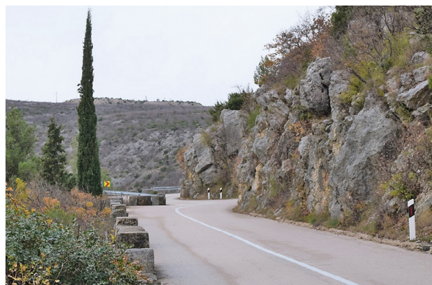
Figure 27: Majstorska Cesta in the Zrmanja River Canyon near Obrovac, cut in by the thick conglomerate strata of the Palaeogene Promina deposits
