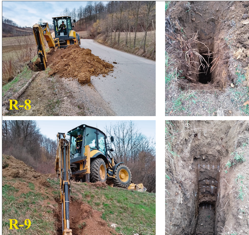
Figure 8: Exploration excavations R-8 and R-9
