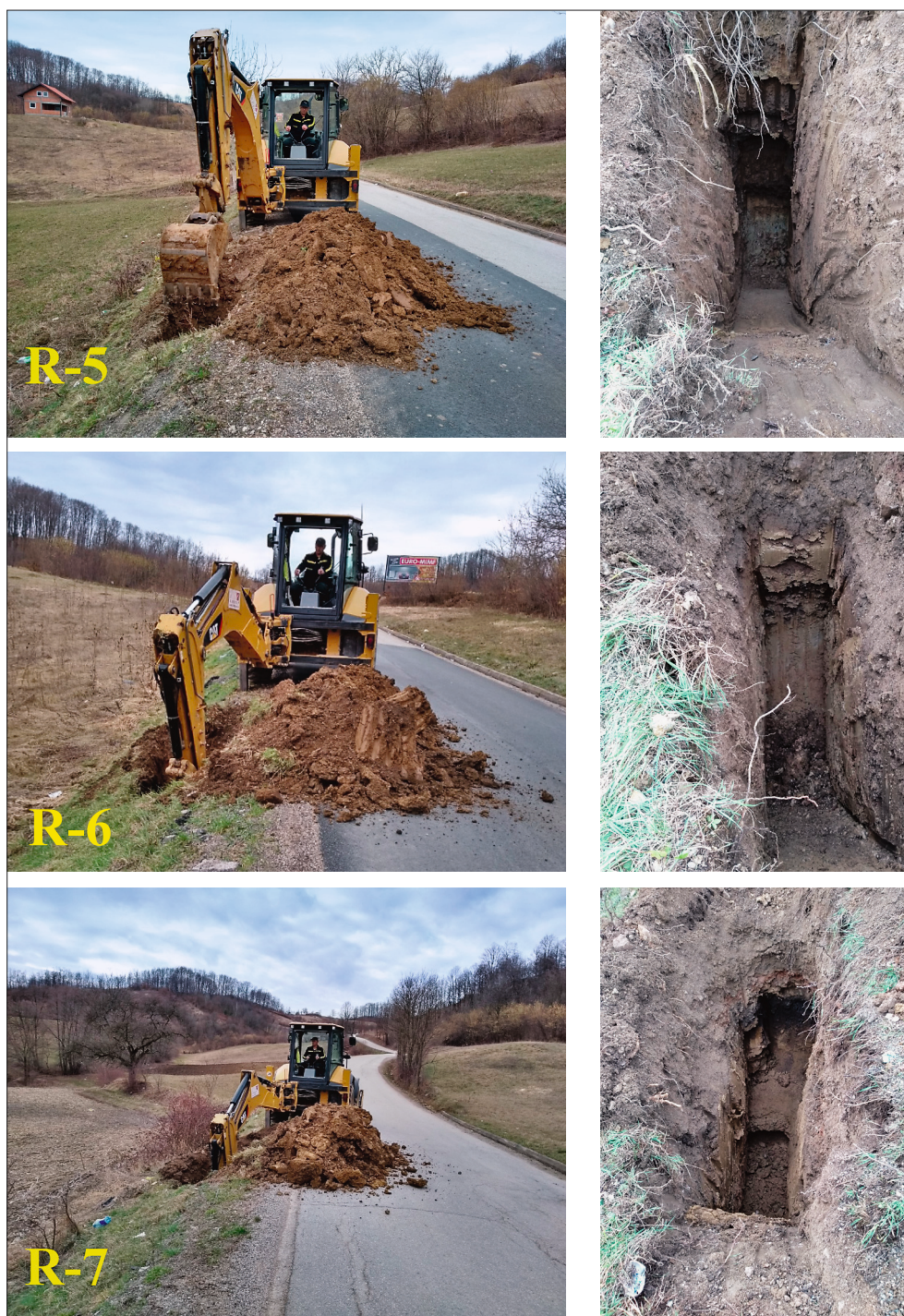
Figure 7: Exploration excavations R-5, R-6 and R-7
