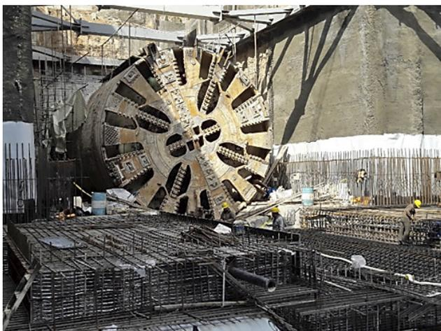
Figure 1: EPB machine used in the Tabriz metro line 2
