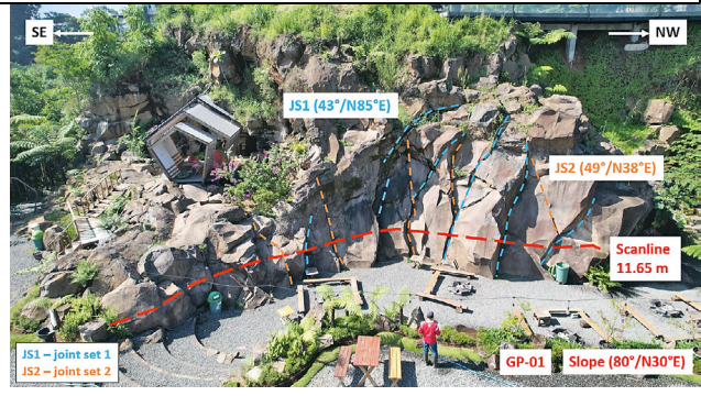
Figure 11: Kinematic analysis results and drone photo of section GP-01
