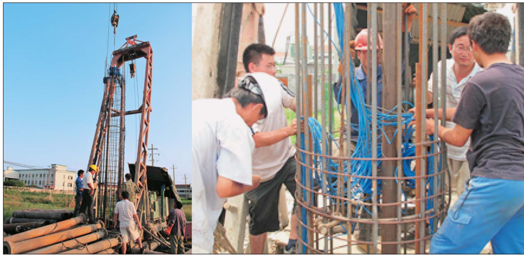
Figure 3: Test pile construction
