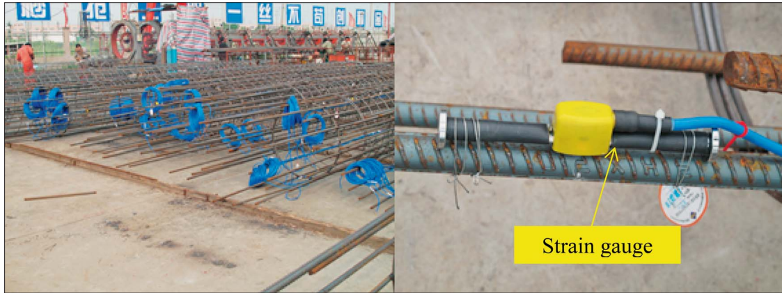
Figure 2: Installation of strain gauges on the test pile
