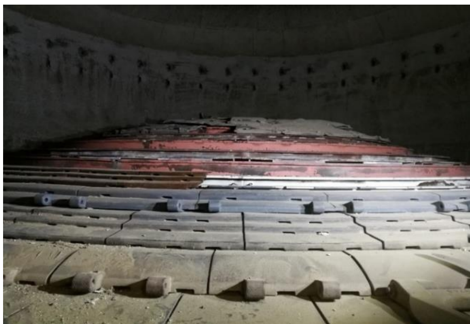
Figure 2. The firebox in the overhaul phase
