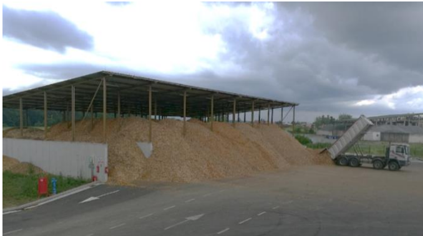
Figure 1. Wood chips warehouse
