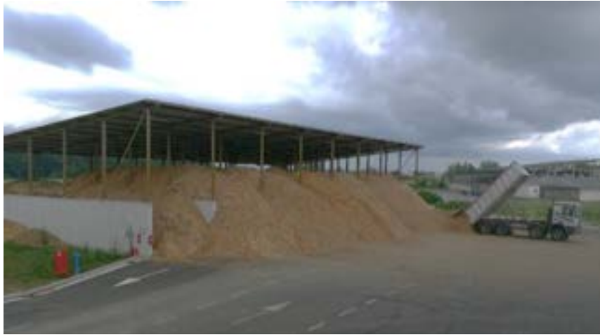
Figure 1. Wood chips warehouse
