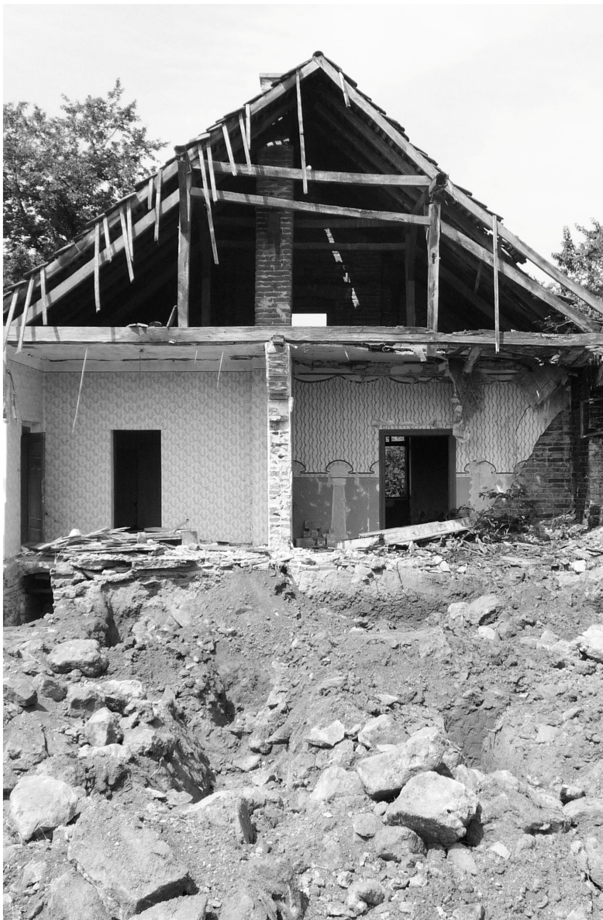
Photo 091. Demolished house / Srušena kuća
