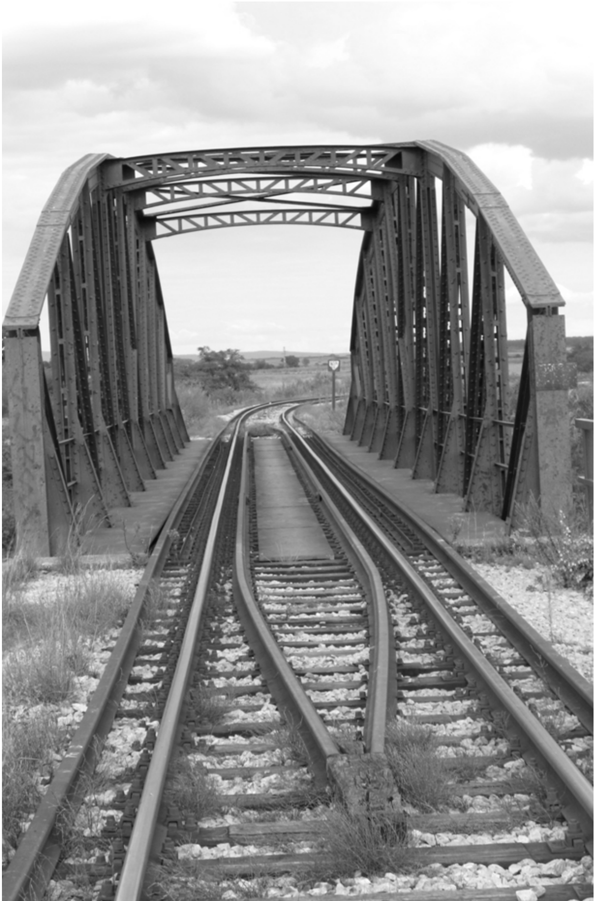
Photo 166. Orłjawa bridge / Most na Orłjavi
