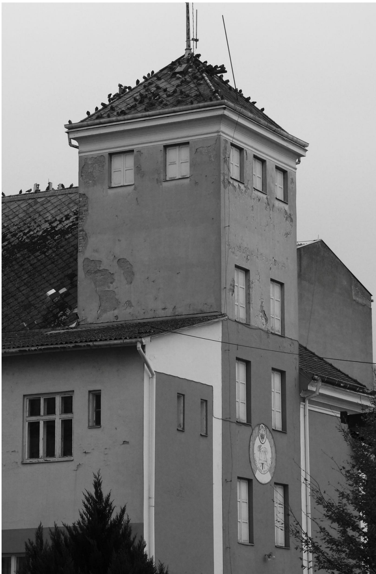
Photo 022. Firehouse / Vatrogasni dom
